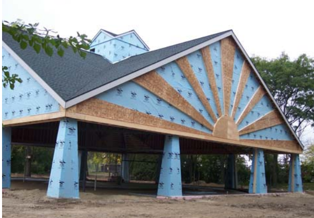
The year-round building that will house the Carousel
